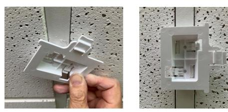
Plug in the network cable or other port cables and slide the unit onto the ceiling bracket until the latch clicks in place.
